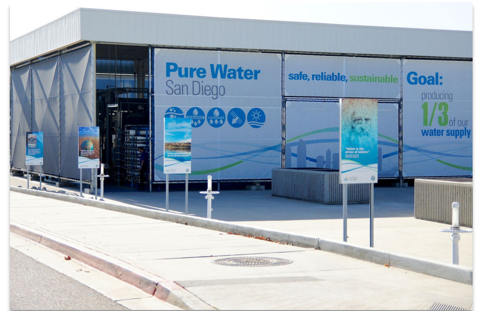
City of San Diego Pure Water Demonstration Facility Operational since 2011
