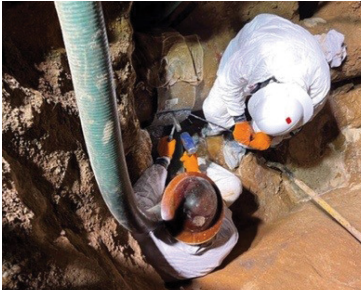
PWD construction crew don hazmat suits while working on a leak involving asbestos concrete pipes
