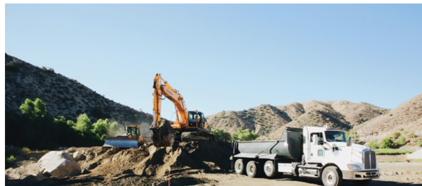
Contractors start removing sediment at the Littlerock Reservoir
