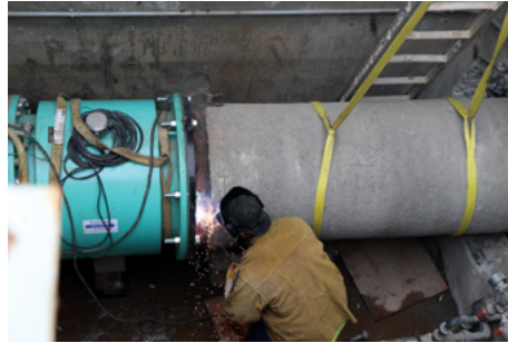
PWD construction crew working on repairs.
