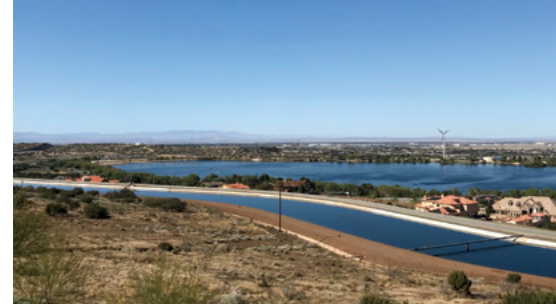
Aerial view of the California Aqueduct, Lake Palmdale and the Leslie O. Carter Water Treatment Plant.
