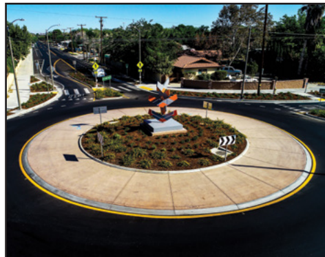
Lancaster Boulevard received street improvements that included the addition of two roundabouts, one at 15th Street East and the other at 15th Street West.
